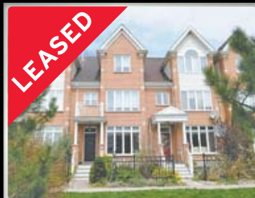
RIVER OAKS $1,850/MONTH Fabulous three storey TH finished on all levels! Newer broadloom, eat-in kitchen, second floor laundry, third floor master w/a vaulted ceiling & walk-out to deck.
